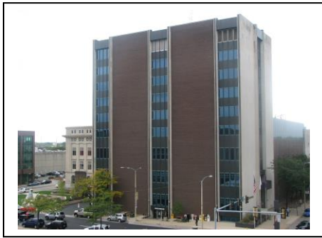
Winnebago County Courthouse 400 West State Street Rockford, Illinois 61101
