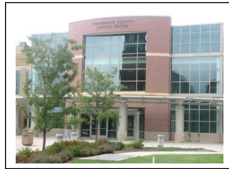
Winnebago County Criminal Justice Center 650 West State Street Rockford, Illinois 61102
